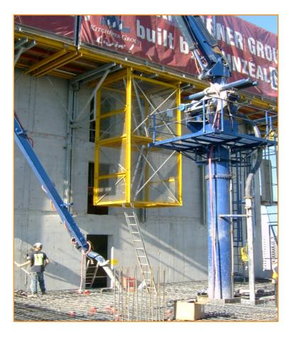
Construction of a 33 storey apartment building for Mainzeal Construction. All Insitu construction using Highrise supplied Boxer Jumpform System and a Ischebeck Flooring Falsework System.
